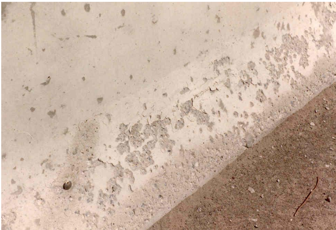
FIGURE 4 Example of Medium Scaling
