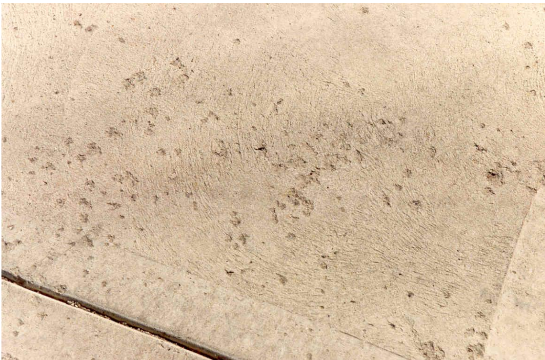
FIGURE 2 Example of Light Scaling
