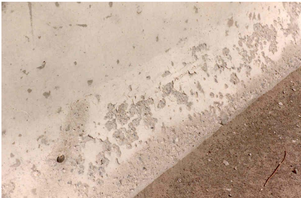
FIGURE 4 Example of Medium Scaling
