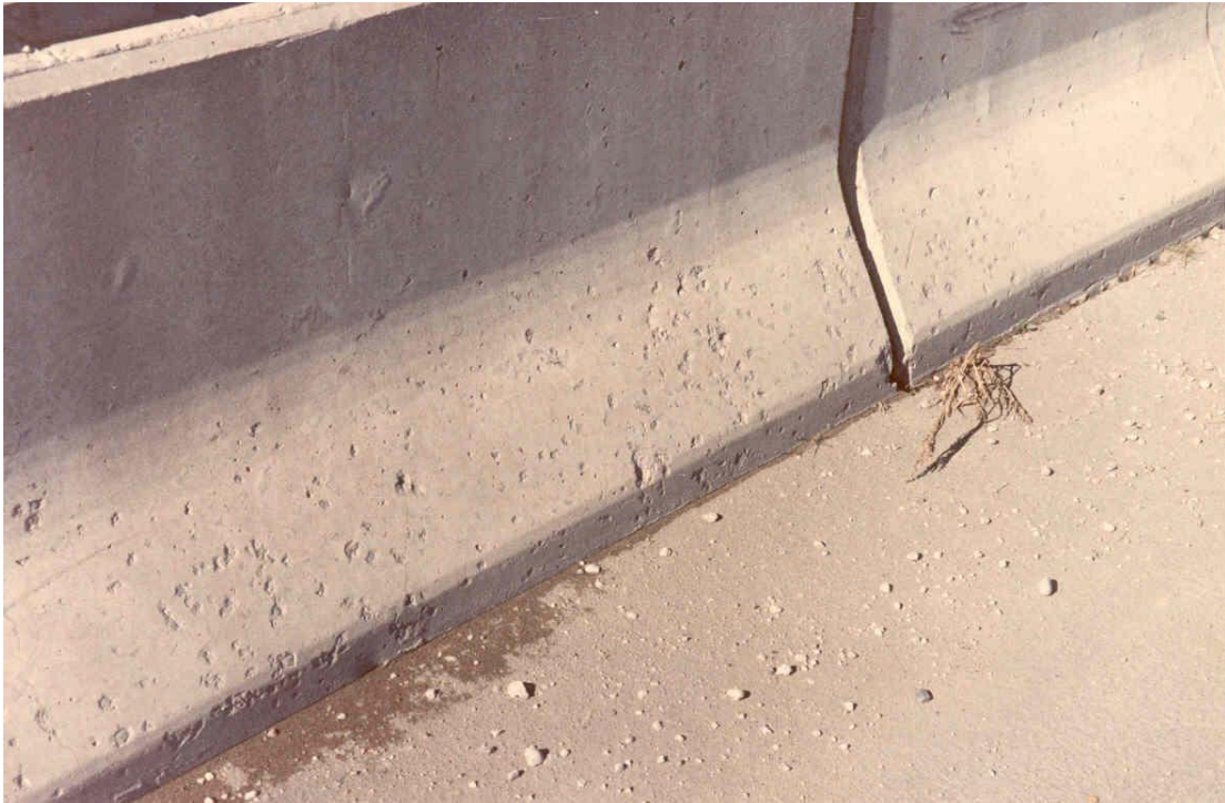
FIGURE 2 Example of Light Scaling
