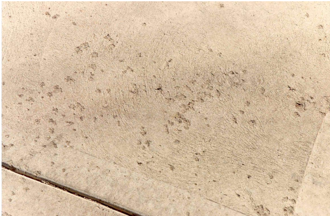
FIGURE 2 Example of Light Scaling
