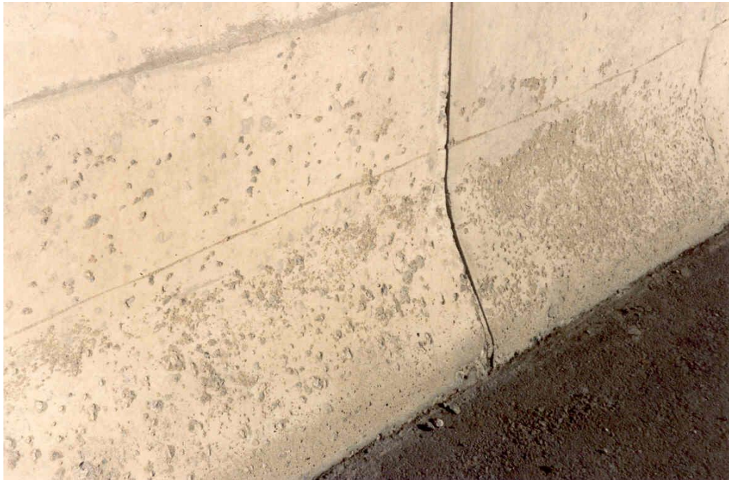
FIGURE 3 Example of Medium Scaling
