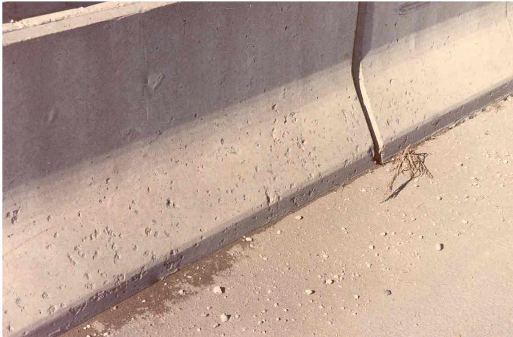
FIGURE 1 Example of Light Scaling
