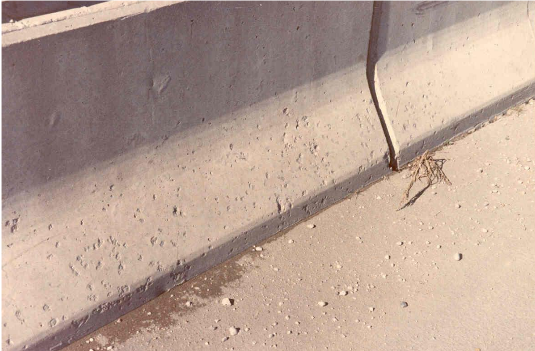
FIGURE 1 Example of Light Scaling
