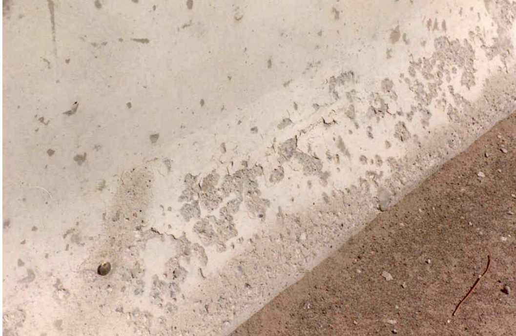
FIGURE 4 Example of Medium Scaling
