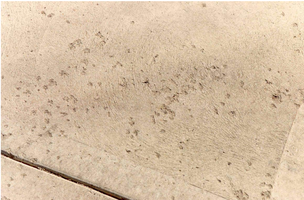
FIGURE 2 Example of Light Scaling
