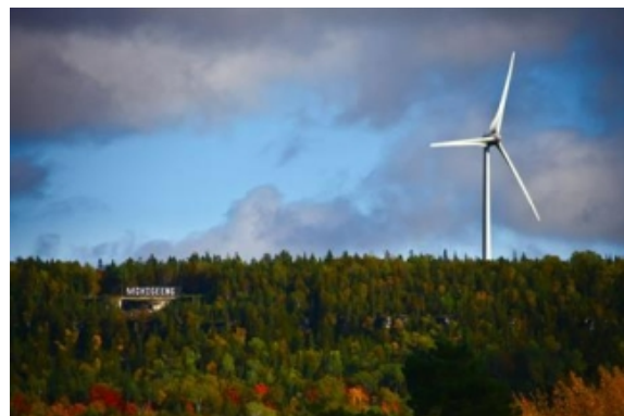
FIT examples: Alderville First Nation's 5 MW solar project (top) & M'Chigeeng First Nation's 4 MW wind project (bottom)
