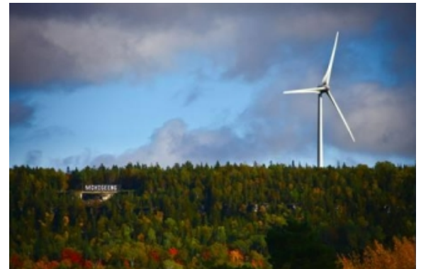
FIT examples: Alderville First Nation's 5 MW solar project (top) & M'Chigeeng First Nation's 4 MW wind project (bottom)
