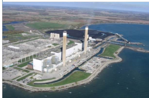
Ontario's largest former coal plant, Nanticoke Generating Station
