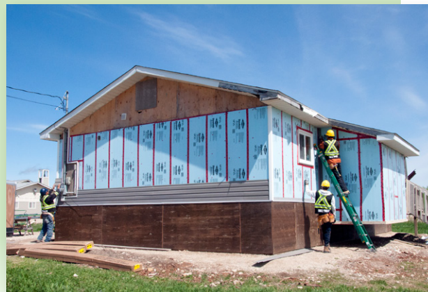
Workers from Conservation on the Coast improve the energy efficiency of a house in the Fort Albany community through the support of Save on Energy incentives.
