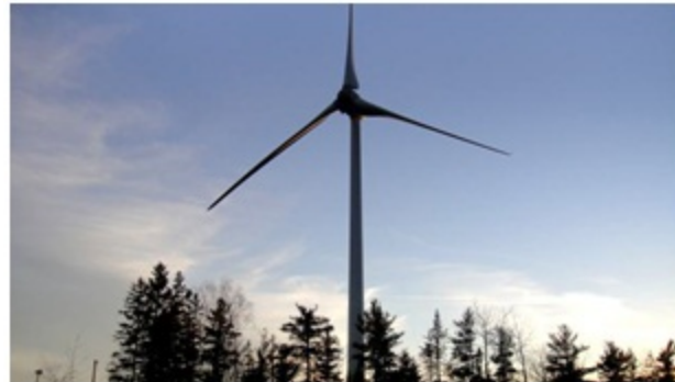
FIT 1 wind project (4 MW), Manitoulin Island, ON
