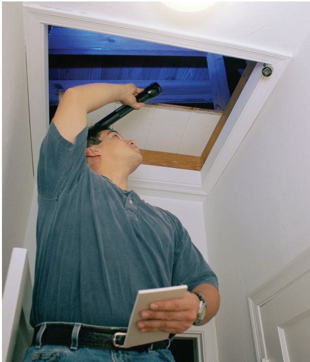
Image 4: Home Energy Audit and Retrofit (source: Enbridge Gas)
