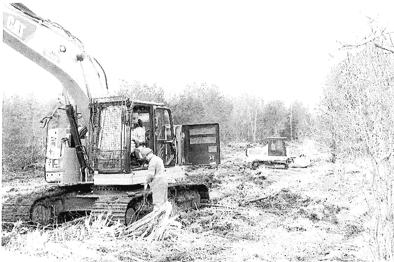
Land clearing at potential turbine site.
