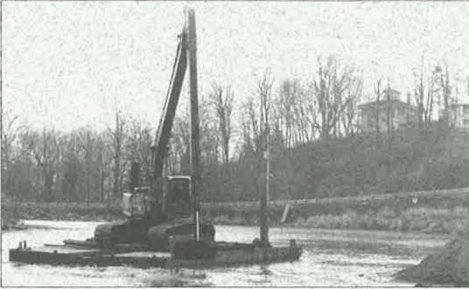
Flood Control Dredging – Port Bruce
