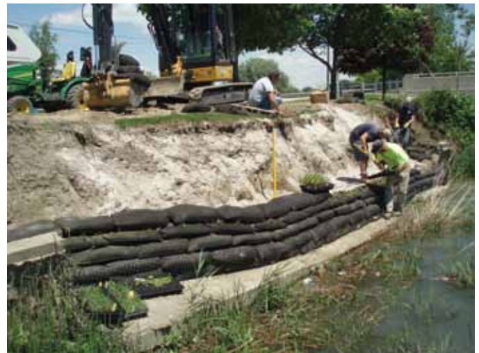
Envirolok bags are used to stabilize a section of eroding bank on the Running Creek dykes in Wallaceburg. The Envirolok bags contain mulch, top soil, and sand which will act as secure anchor and as a growing medium for bank stabilizing vegetation.
