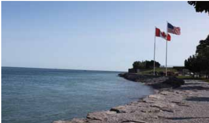
The shore protection work for LAWSS will connect to the protection under the Blue Water Bridge, a popular spot for viewing boats on the St. Clair River.
