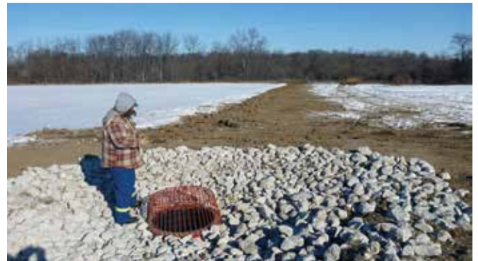
A catch basin was installed to reduce erosion on one of the McKeough upstream properties as part of our program to properly manage our agricultural holdings.
