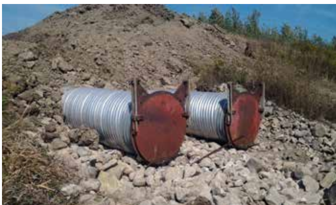
Culverts re-installed to maintain the integrity of the berms along the diversion channel of the McKeough floodway.
