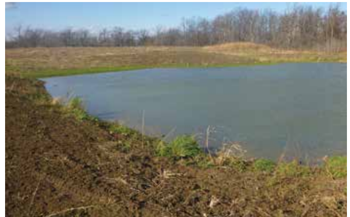
With a little time, this newly constructed wetland will soon be supporting a wide variety of aquatic life, improving habitat and water quality entering local watercourses.
