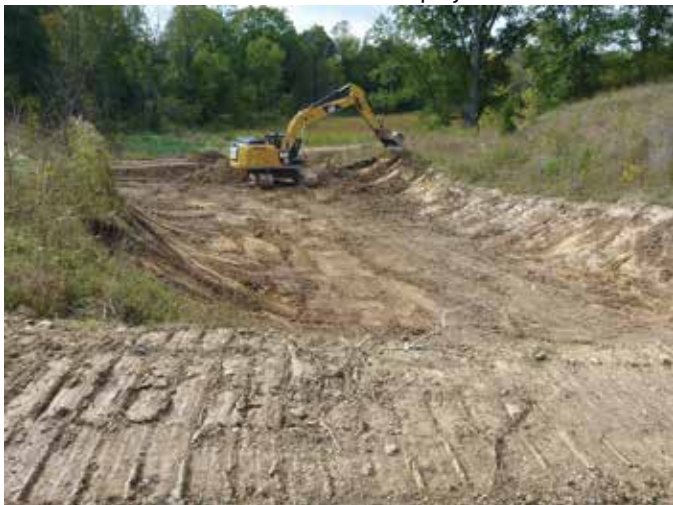
Excavation of a future wetland will create habitat and improve water quality entering nearby watercourses.
