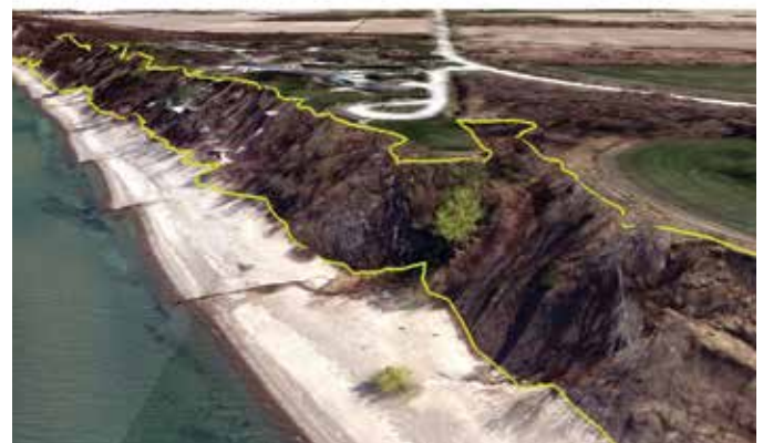
Shoreline Delineation Using 3D Viewing of Digital Aerial Photography
