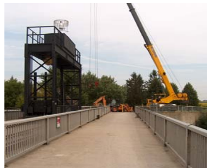
Repairs to the Chesterville Dam
