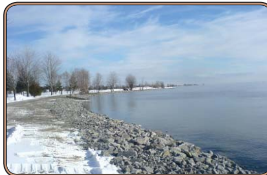
Morrisburg shoreline after shoreline stabilization.
