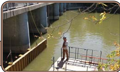
Coffer dam installation.
