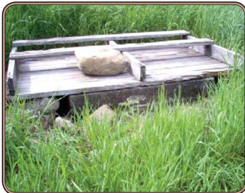
A dug well prior to being decommissioned.
