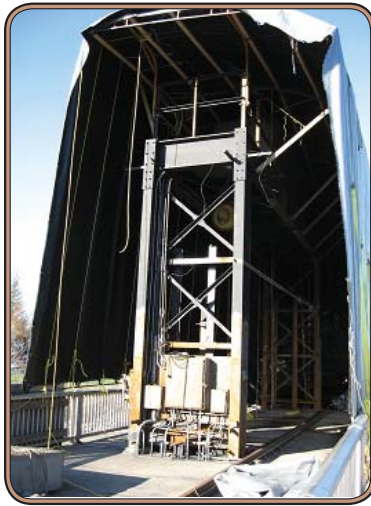
Chesterville dam steel gate.
