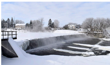
Water Control Structure, South Nation River at Crysler
