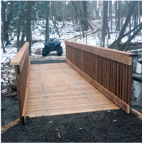
New bridge at J. Henry Tweed CA
