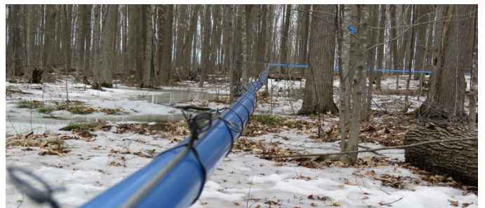
Pipeline through Oschmann Forest in North Dundas
