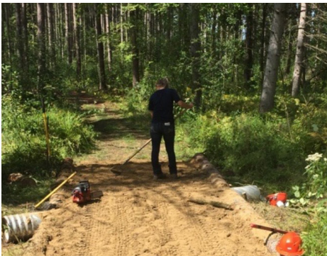
Trails at the Robert Graham Conservation Area in South Dundas were resurfaced and new culverts were installed to help alleviate seasonal flooding.
