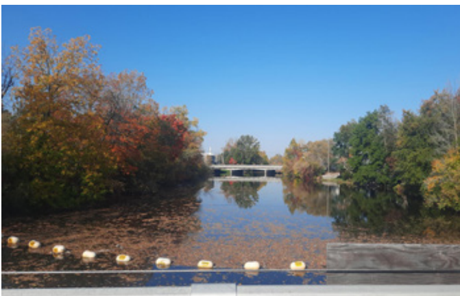
Chesterville Dam, Township of North Dundas
