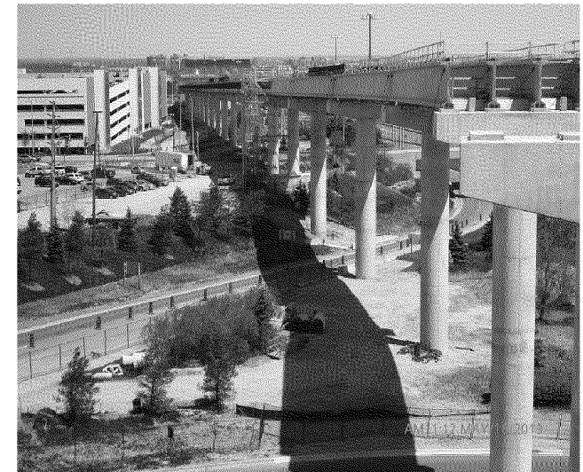
View of spur east of pier 61
