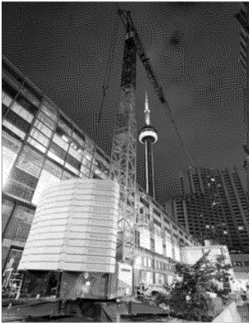
Crane installed at Union Station
