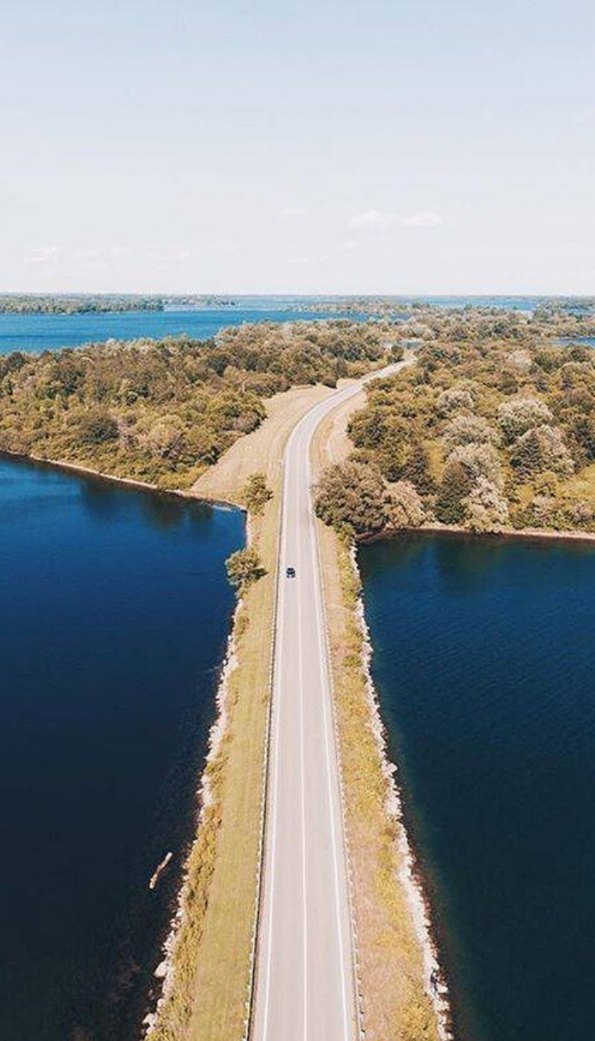
LONG SAULT PARKWAY- SOUTH STORMONT, ON
