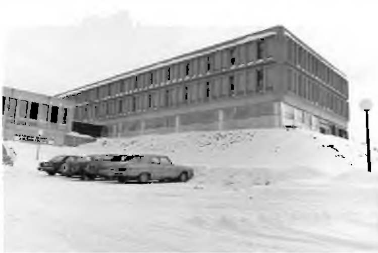
Huntington University during the later construction phase, n.d.
