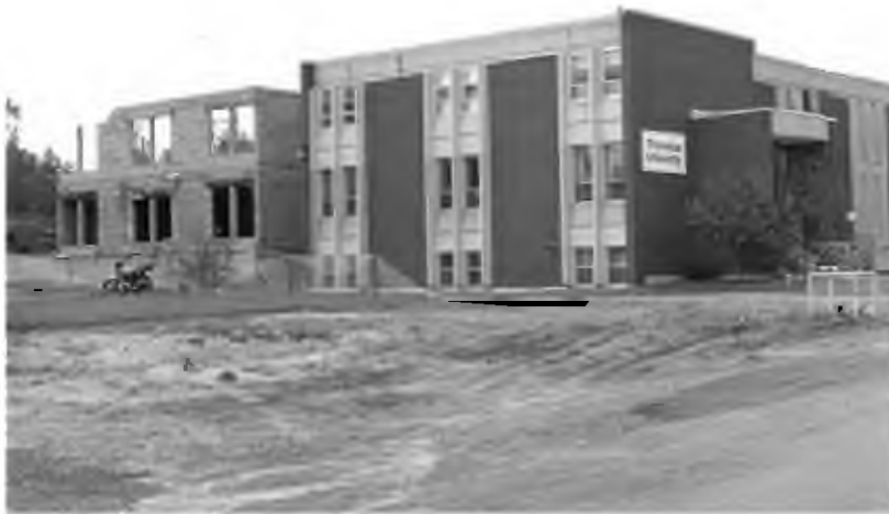
Thorneloe University, Building Extension: July 25, 1990.
