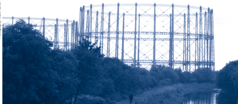
A gas holder that is part of the distribution network in Britain.
