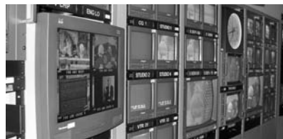
Post-production plant rebuild
