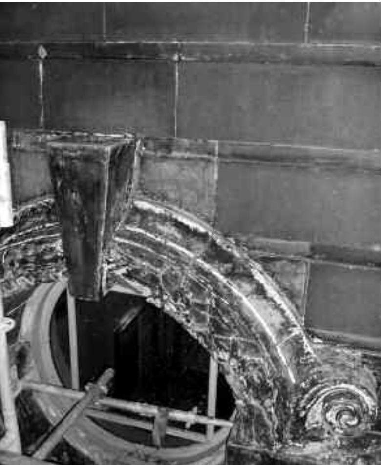
In October 2005, the investigative phase of the façade restoration for the Ontario Heritage Centre in Toronto was completed. The Centre is the headquarters of the Ontario Heritage Trust.
