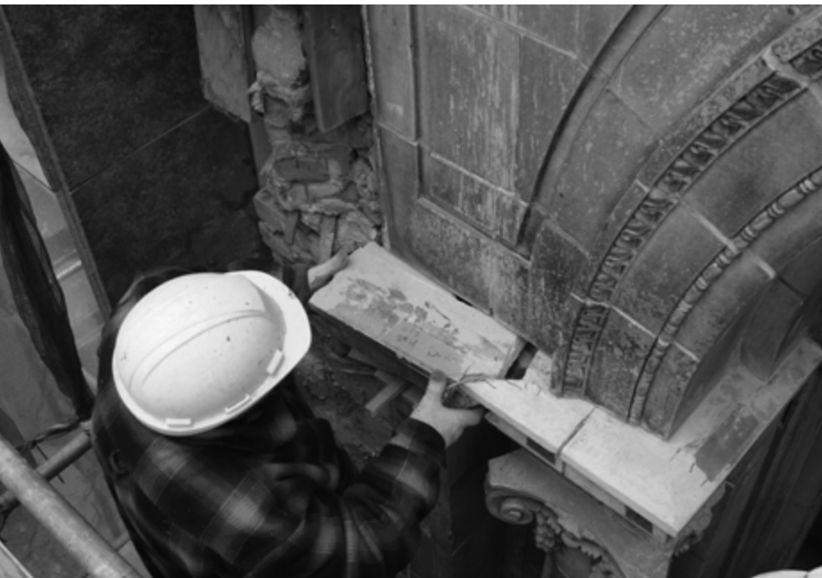
▲ Removal of a terra cotta unit for replication, Elgin and Winter Garden Theatre Centre, Toronto
