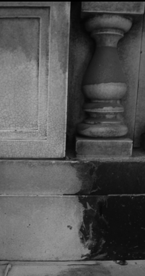
▼ Test cleaning of terra cotta exhibiting surface crazing, Elgin and Winter Garden Theatre Centre
