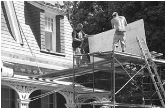
Replacing the cedar roof at the Ashbridge Estate in Toronto
