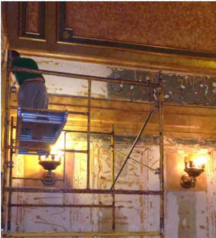
Restoration of decorative wall panels in the Elgin and Winter Garden Theatre Centre; before and after.
