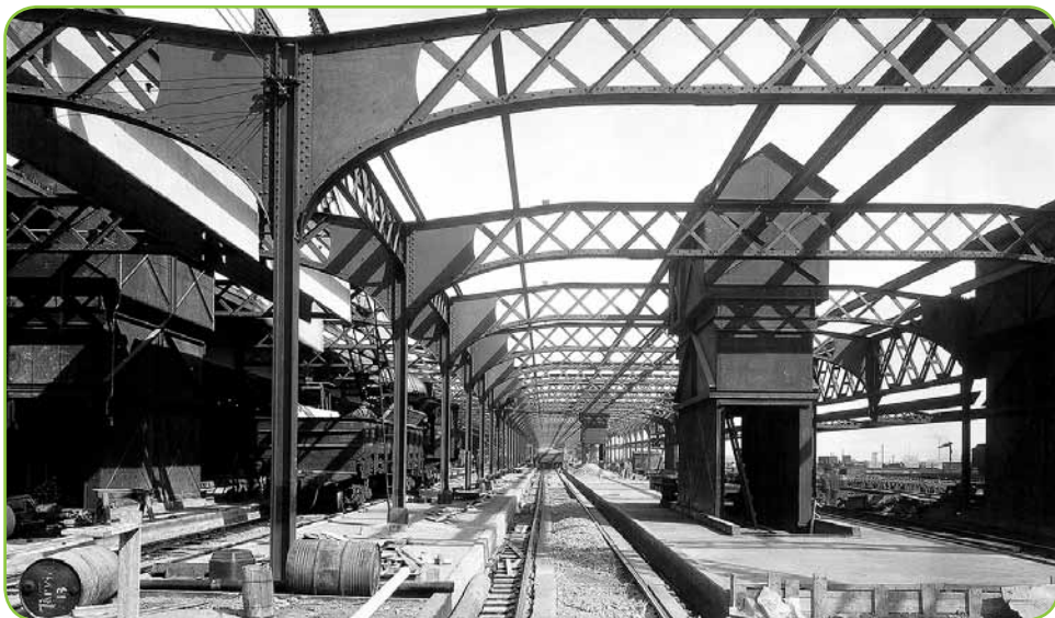
Early construction at Union Station.
