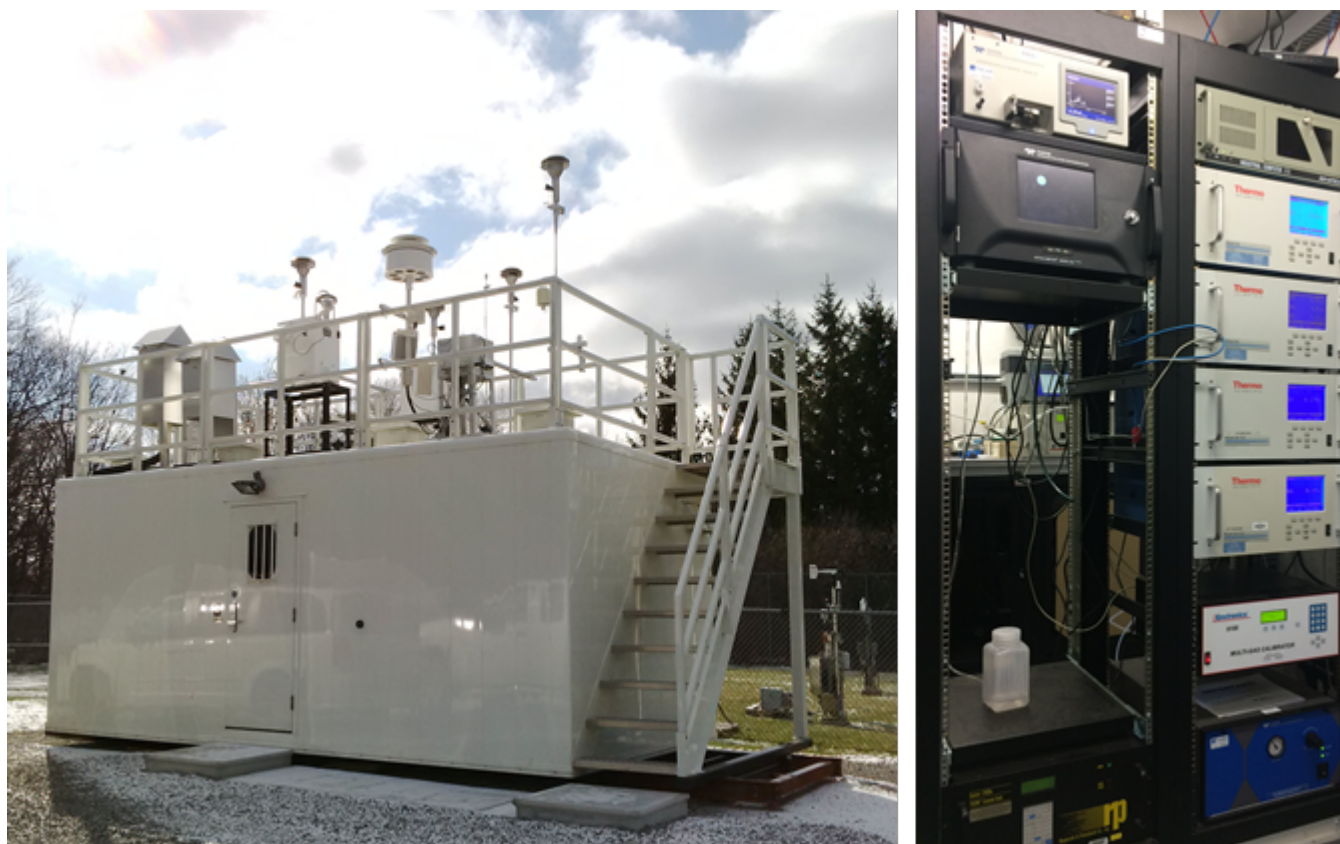
Two photographs showing the exterior (left) and interior (right) of the Toronto North Air Quality Health Index Station.
