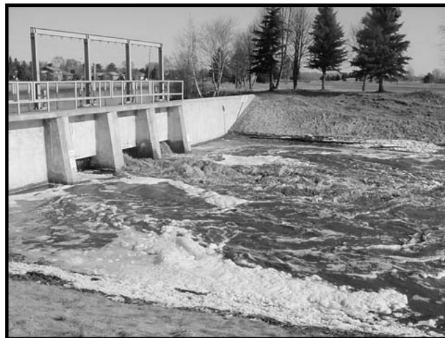
Above: During the Easter flood event, the Diversion Structure restricted flows down the Neebing River. The Diversion Channel carried the excess flow, which ran more than a metre deep.
