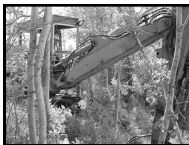
Left: Drilling equipment was used to install soil nails for bank stability testing.
