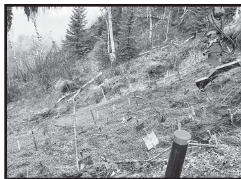
Above and Below: Long steel bars driven deep into the ground will stabilize the river bank at five sites along Victor St.
