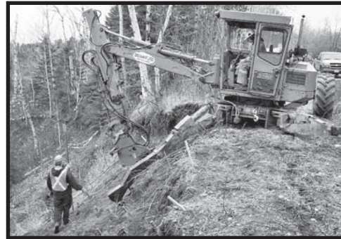
Above and Below: Long steel bars driven deep into the ground will stabilize the river bank at five sites along Victor St.
