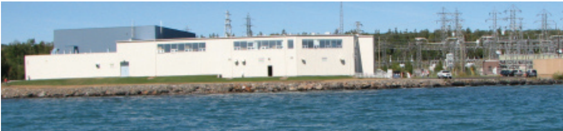
Bare Point Water Treatment Plant
