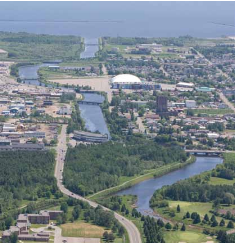
The Neebing-McIntyre Floodway in the Intercity Area
