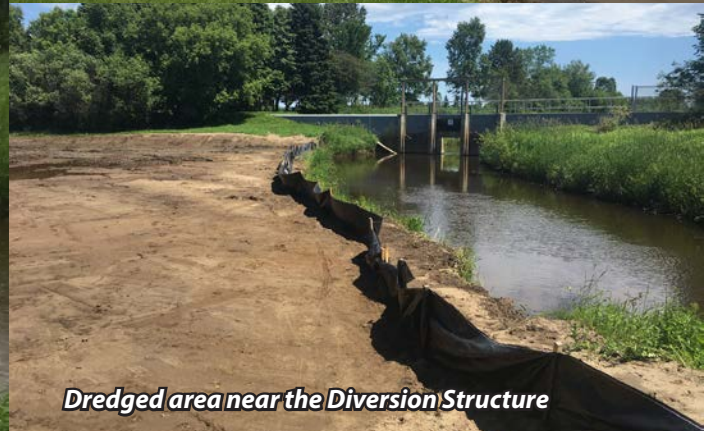
Sedimentation dredging of the Diversion Channel
