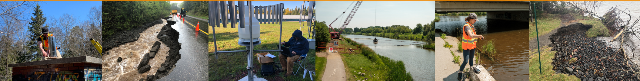
Photos (left to right): spring tipping bucket inspections; washout on Highway 588 during June flooding event on Whitefish River; maintenance of weather station in Township of Dorion; maintenance sediment dredging on the Floodway; testing turbidity along the Floodway; erosion at Mission Island Marsh.
