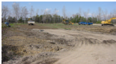
Road construction began at the Chatham-Kent Children's Safety Village located at C.M. Wilson Conservation Area.
