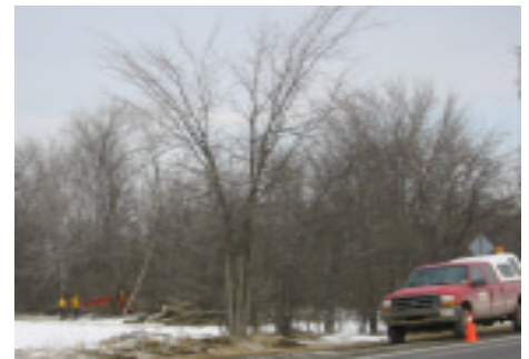
Approximately 90,000 ash trees were cut and mulched in the ash free zone.
