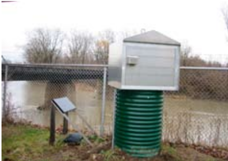
In 2005, the LTVCA received 100% funding from Environment Canada and the Ministry of Natural Resources to undertake upgrades at two of our existing stream gauge locations. The installations of a new roof on the McGregor Creek stream gauging station, a weir at the McGregor Creek stream gauging station and a new housing for the Chatham water level monitoring station, cost a total of $20,000.
