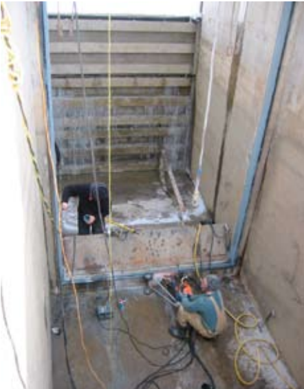
Repairs to McGregor Creek Dam included replacing hinges with stronger continuous strip hinges, modifying the hoist mechanism to reduce the lifting forces on the hinges and modifying the limit switches to detect when the gates are closed.
