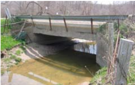
This bridge will be replaced with a similar structure like an open bottom culvert. This type of replacement is preferred as it allows free fish passage without disturbing the bed of the system, allowing for a low flow channel within the culvert section.
