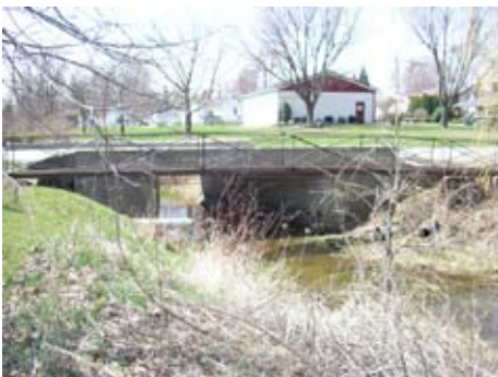
Surveys of road bridges will determine flood plain areas in rural areas.
