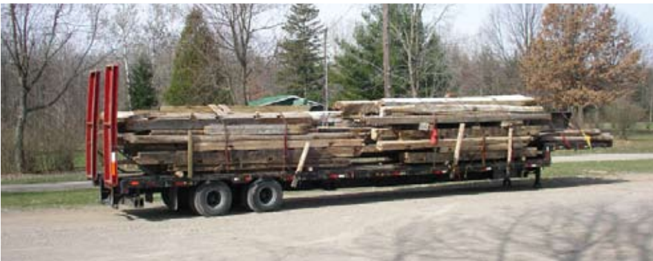
Old barn timbers were saved and transported from London to Longwoods to be used to replace rotting timbers in the cabins.
