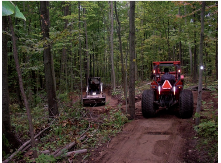
Work began in August with the removal of hazard trees and the blazing of the new section of the trail.
