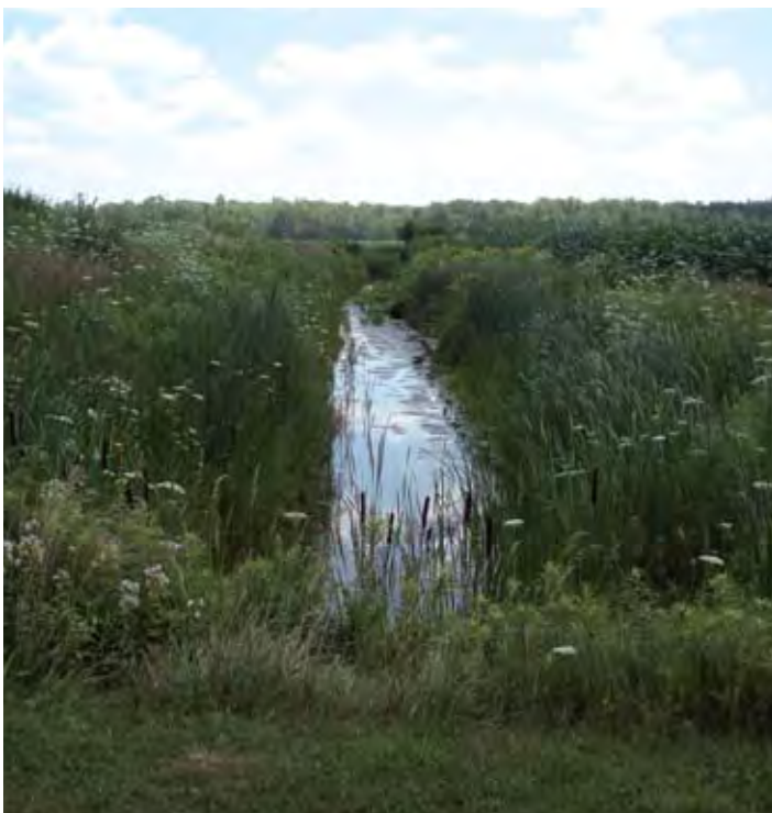
Municipal Drain maintenance was undertaken, which protected side bank vegetation. This helped to retain bank stability and habitat value.
