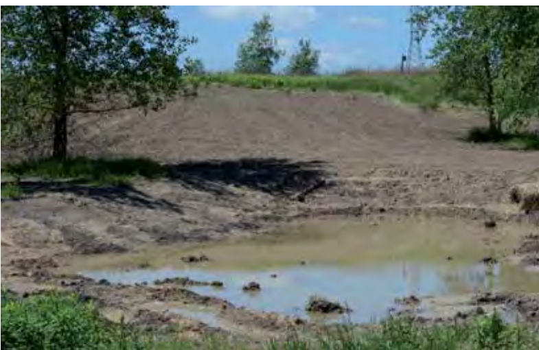
Two ponds were excavated to create a wetland complex at the Diversion Channel Conservation Area . Tree and wetland plant species were planted, and phragmites control was undertaken.
