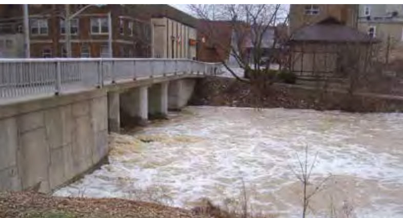
The 6th Street Backwater Dam and Pumping Station at the mouth of McGregor Creek in Chatham, operated during the mid-April flood.
