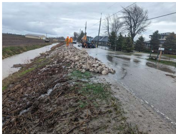
Erie Shore Drive road flooding, April 17, 2023
