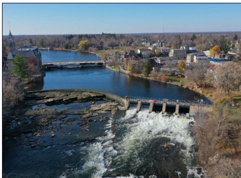
Aerial view of the Carleton Place Dam
