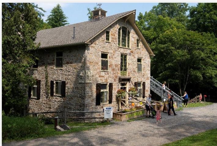
Mill of Kintail Museum, new roof
