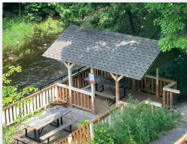
Mill of Kintail lookout, new roof
