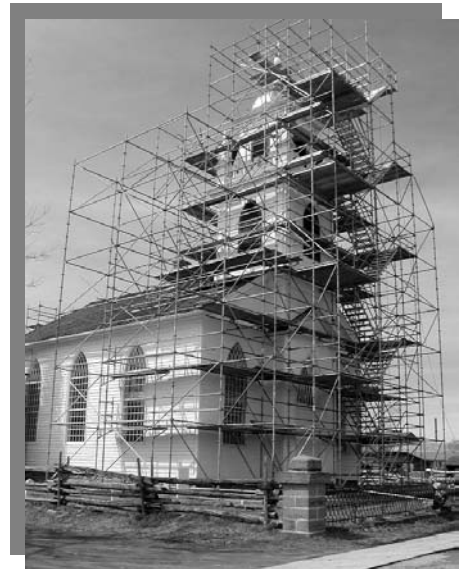
Repairs underway at Christ Church (Upper Canada Village).
